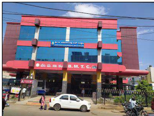
Figure 2 Photo of Yelahanka Old town Bus Station
